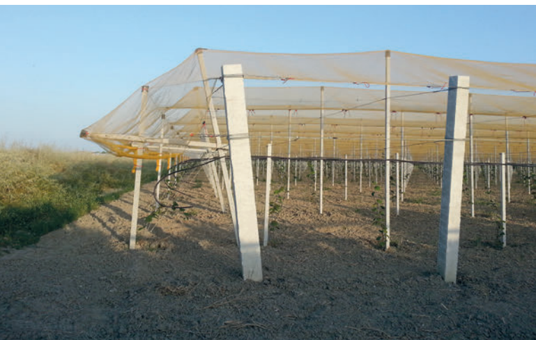
The main structural component of the trellis system is the concrete post.
