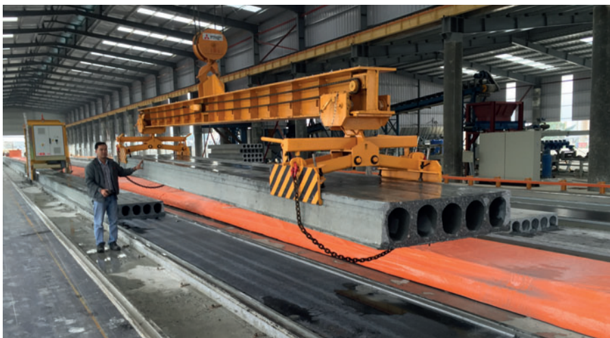
Lifting of the hollow core slab from the production bed
