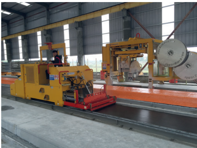
Multi-function cleaning machine during the preparation of the production bed
