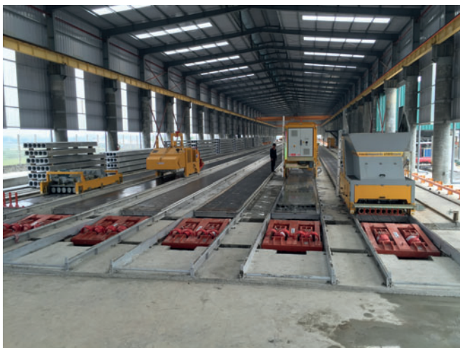
General view of the new production plant of hollow core slabs in the city of Hanoi
