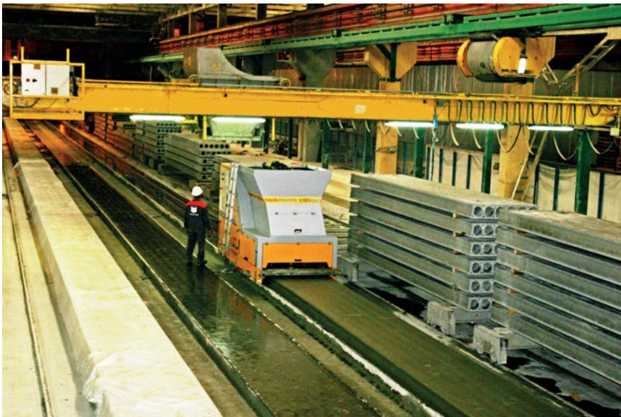
JBI-5 modernized its existing plant and installed a hollow core slab production line for production of 1200 mm slabs.
