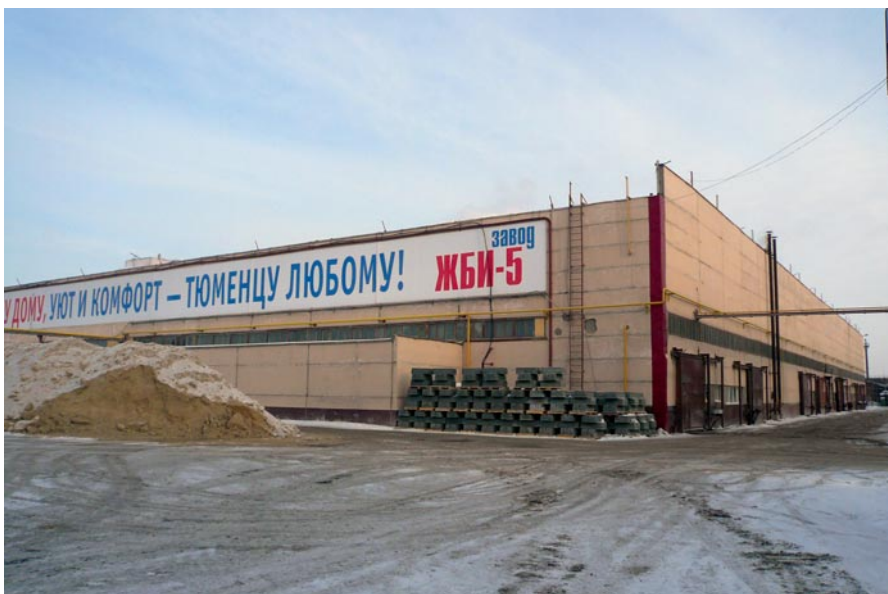
JBI-5 became first Russian partner of Nordimpianti in the city of Tyumen and continues to choose Nordimpianti as its main supplier.
